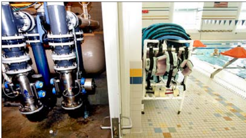
ETS chambers installed at Utah Pool
